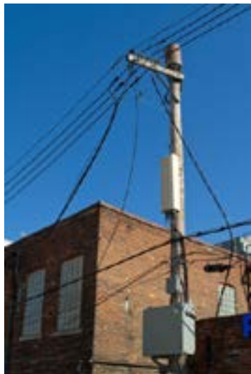
FlexWave Prism DAS co-located in the telecom right-of-way
